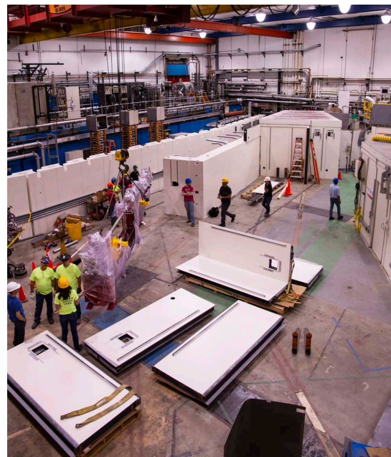
Top Left: CHESS's Ernie Fontes, left, inspects the pre-fabricated hutch at the ADC facility. This hutch was later disassembled and transported to Wilson Lab for a seemingly quick assembly, top right.
